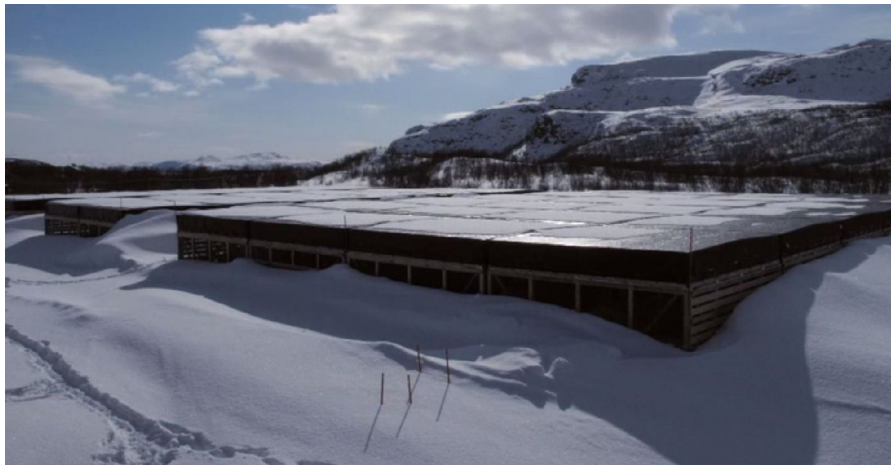
High-Band Antenna (HBA) array 51m x 31 m 48 tiles 110-270 MHz
